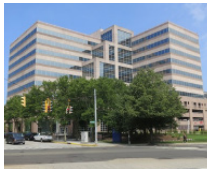
750 Washington Blvd., Stamford
